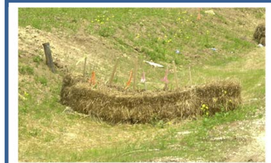
Example of a straw bale ditch check to prevent erosion.
