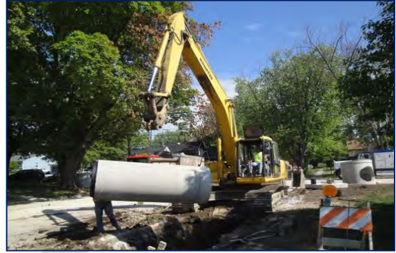
Figure 6. Typical Storm Sewer Construction
