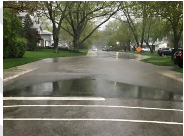
Figure 13. Inundation at Central Avenue (Birchwood Avenue Intersection)
