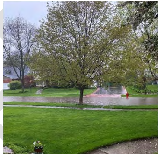
Figure 19. Inundation at Shannon Road
