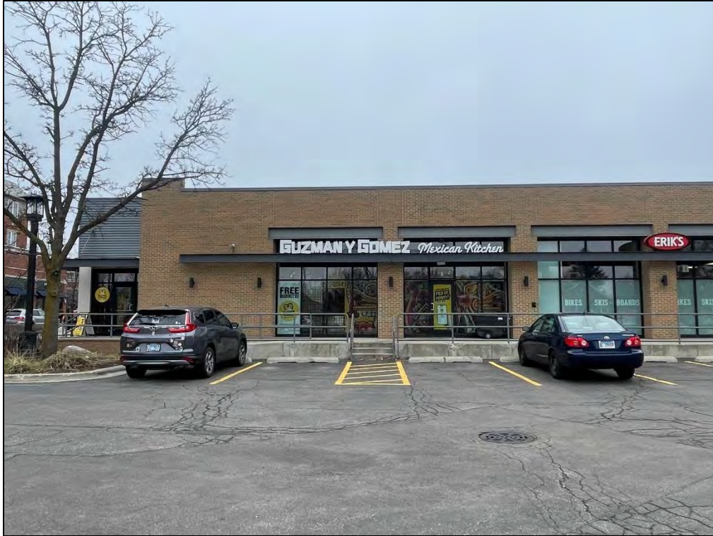
Existing East Wall Sign
