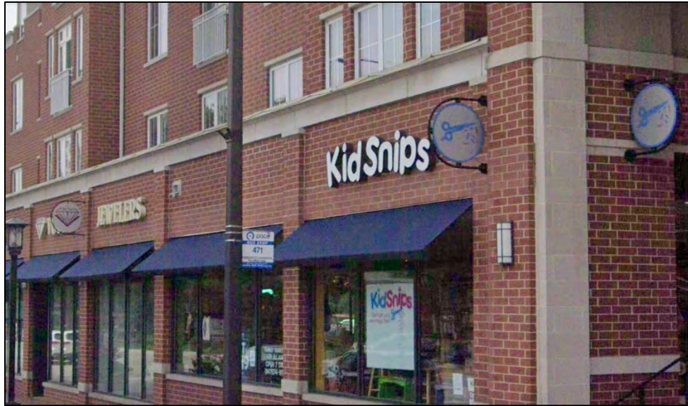
Existing Blade Signs at Deerfield Village Centre
