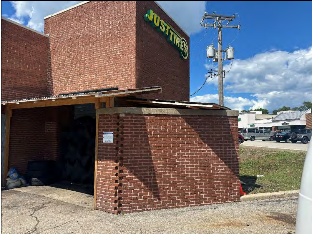
Just Tires Building Alteration to be Removed
