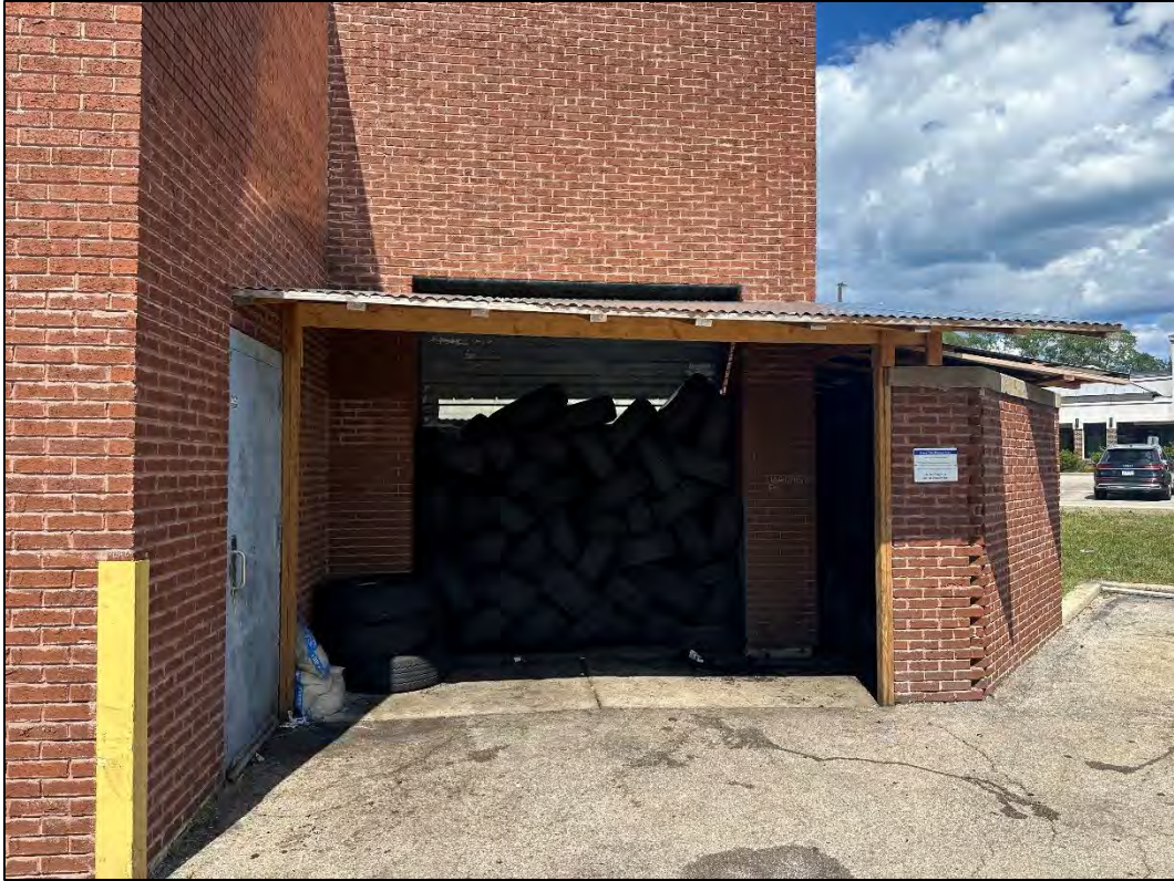
Just Tires Building Alteration to be Removed
