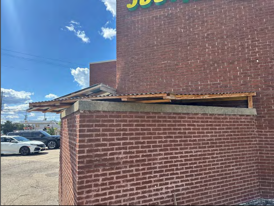
Just Tires Building Alteration to be Removed
